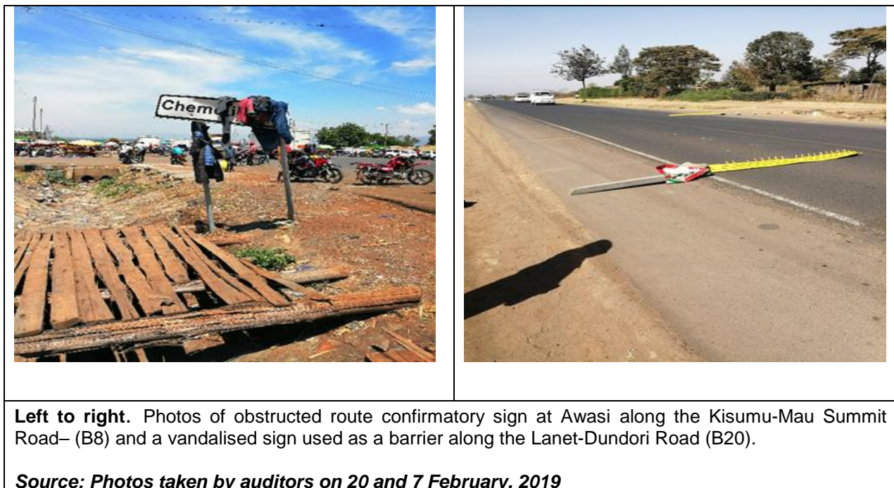
Figure 4: Inappropriate use of Road Furniture by the Public
