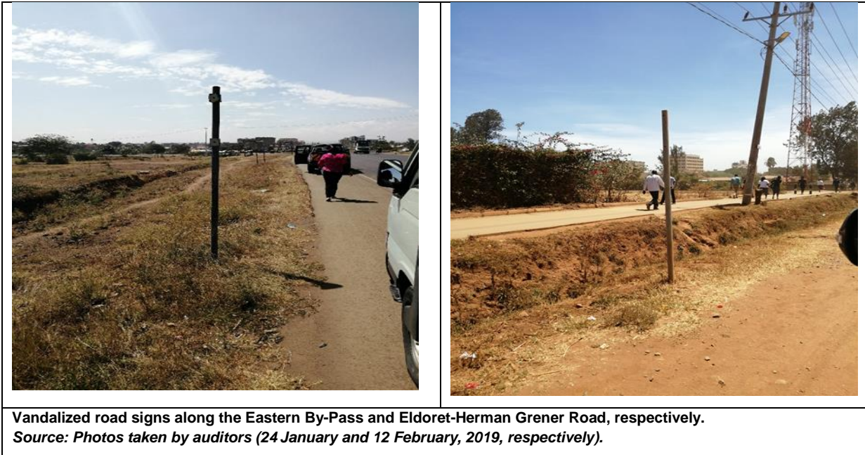
Figure 6: Vandalised Road Furniture
