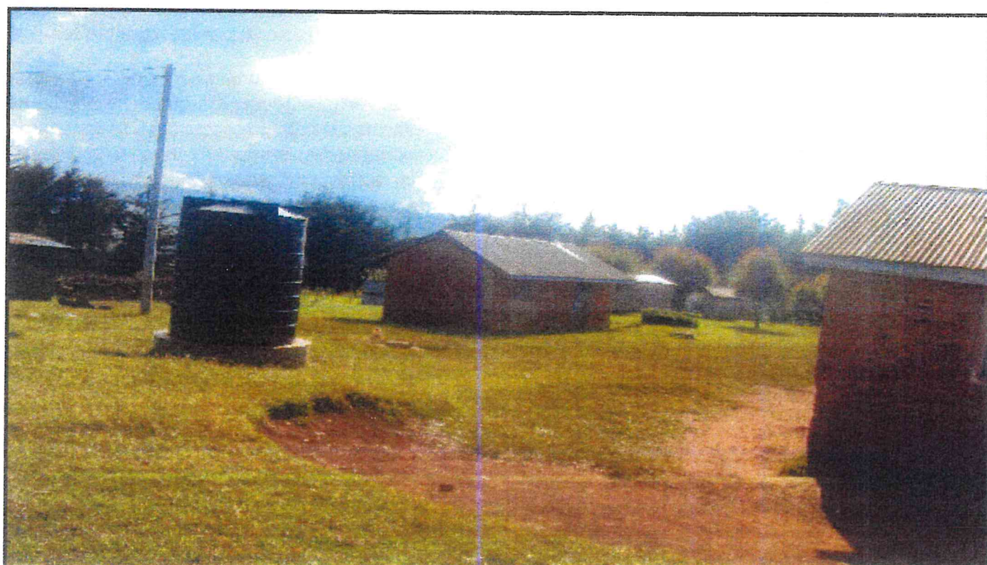
Plate 1: Water tank taller than the roof and against gravitational flow. Note: No guttering system installed at Skyline Primary School
