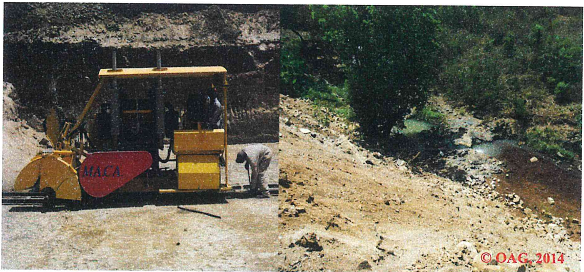
Picture 4: Quarrying Activity in Mitunguu, Meru
