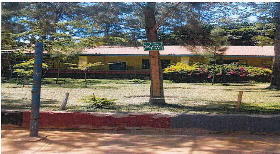
Source: OAG Staff physical verification of a fire assembly point in a sampled school
