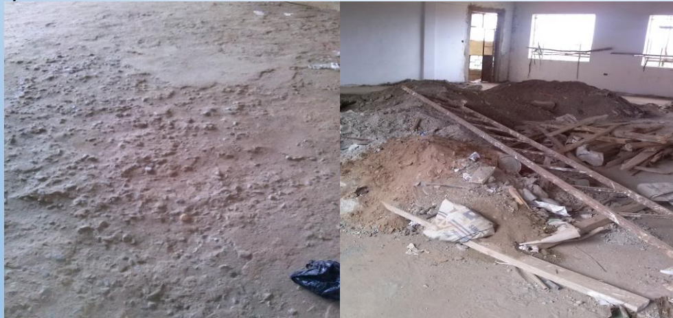
Photo showing status of the project
