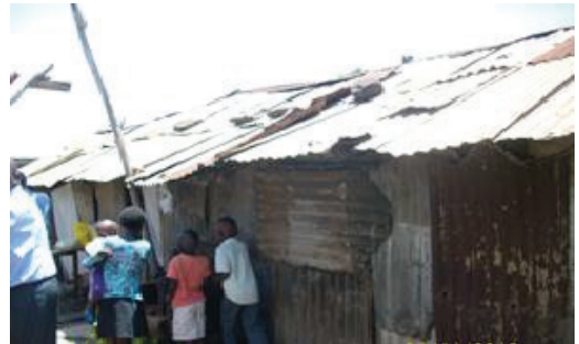
v) Iron sheet house (Nairobi Remand)
