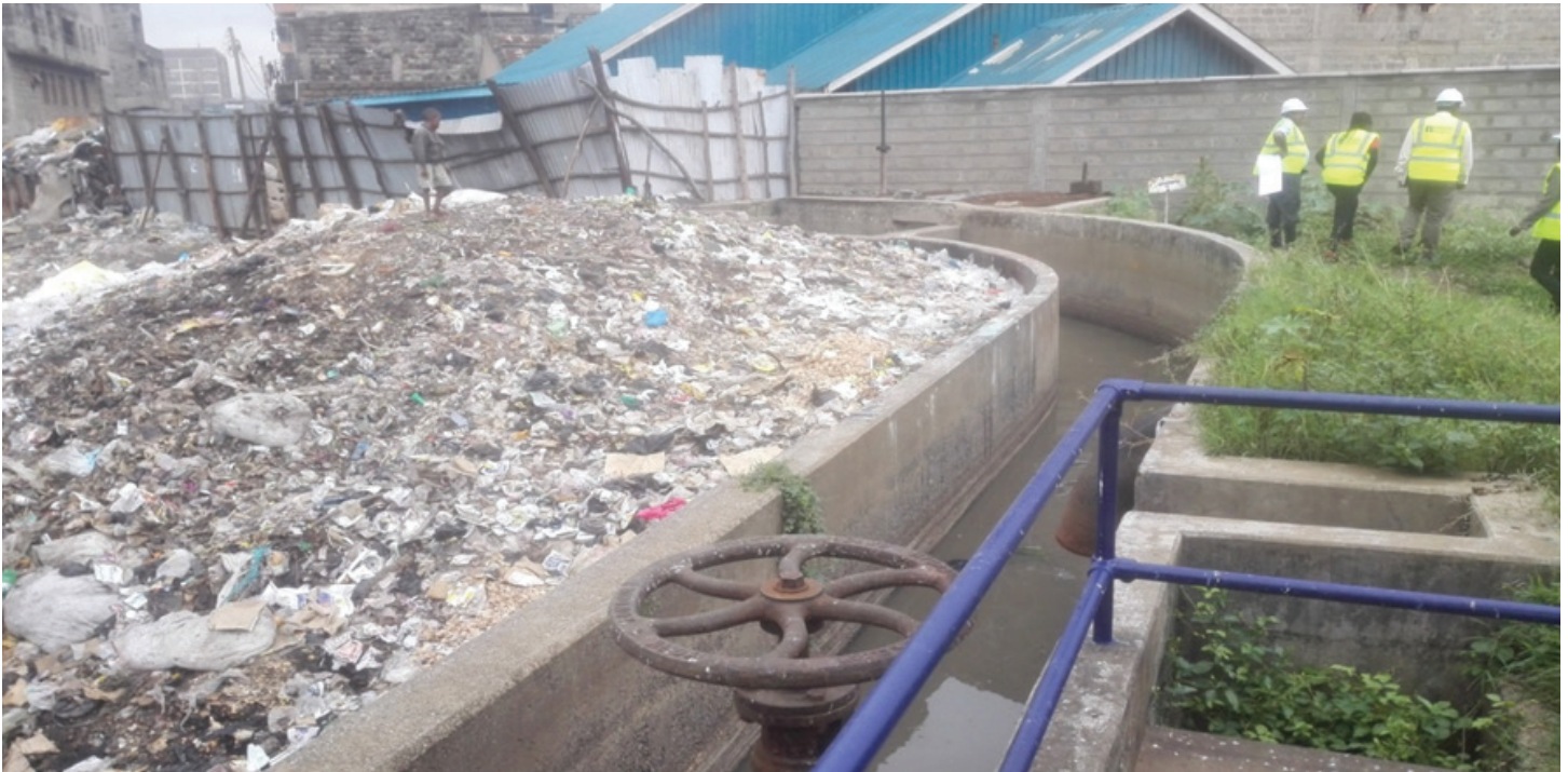
Plate 5: Human encroachment into Kariobangi Waste Water Treatment Plant
